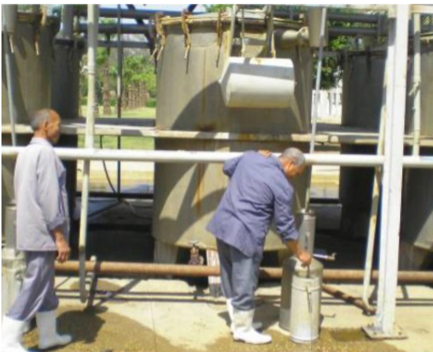
Chamomile distillation facility Kato Aromatics
