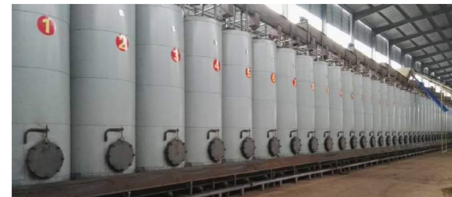
DISTILLATION EQUIPMENT for crude oil from sawdust
