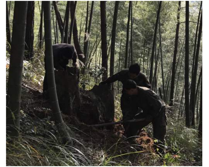
DIGGING OUT THE ROOTS
