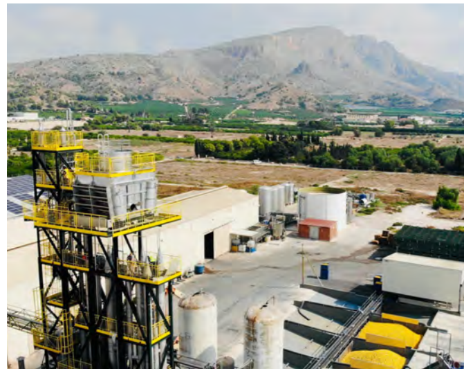
1- RIVERBEND ESPAÑA, S.A. FACILITIES
