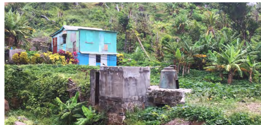
1. A DAMAGED DISTILLERY
